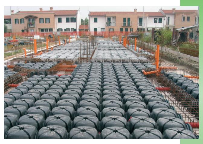
Plastic dome concrete forming system for areated floors
